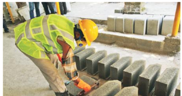
A worker demoulding LC 3 kerb-stones in Jhansi
