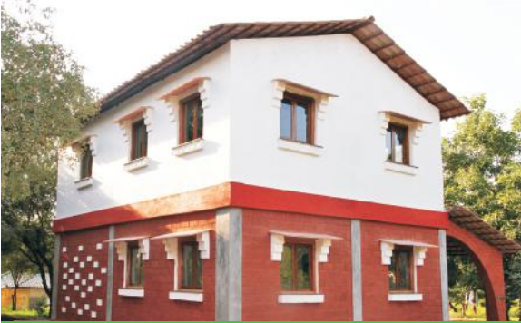
The LC 3 building in Jhansi built using the first batches of LC 3 produced in Jhansi
