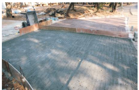
Road segments made using LC 3 in Chennai
