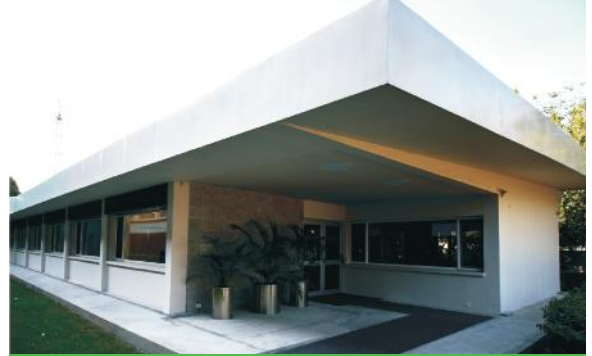
The SDC building at the Swiss Embassy in Delhi having AAC blocks made of LC 3
